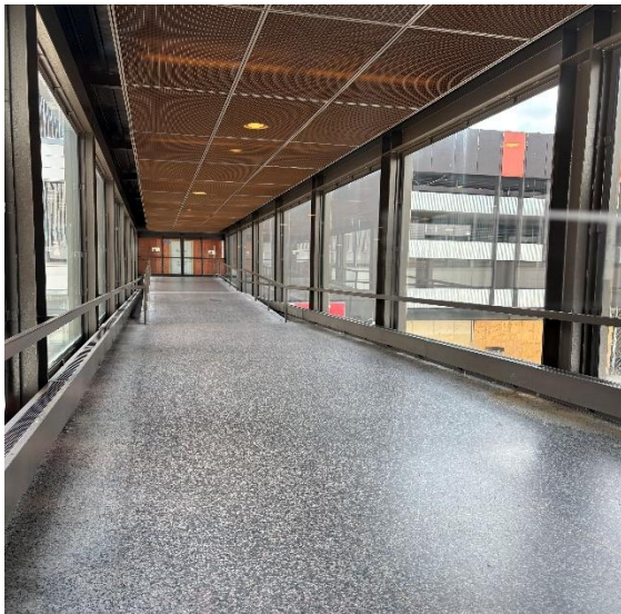
Interior view of Bridge 21
