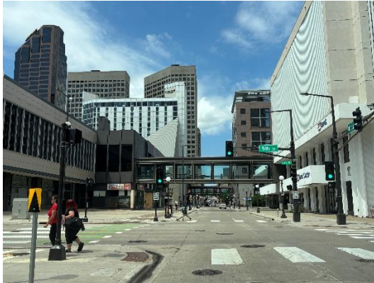
Minnesota Street exterior view of skyways: Bridge 21 & Bridge 11
